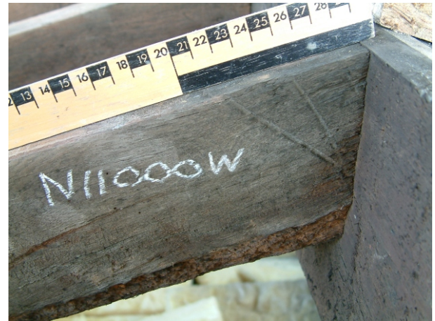
B: Truncated race knife mark \diagdown on common rafter 2R7
