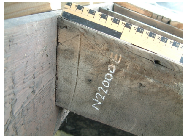
D: Race knife mark \diagup on common rafter 5R7
