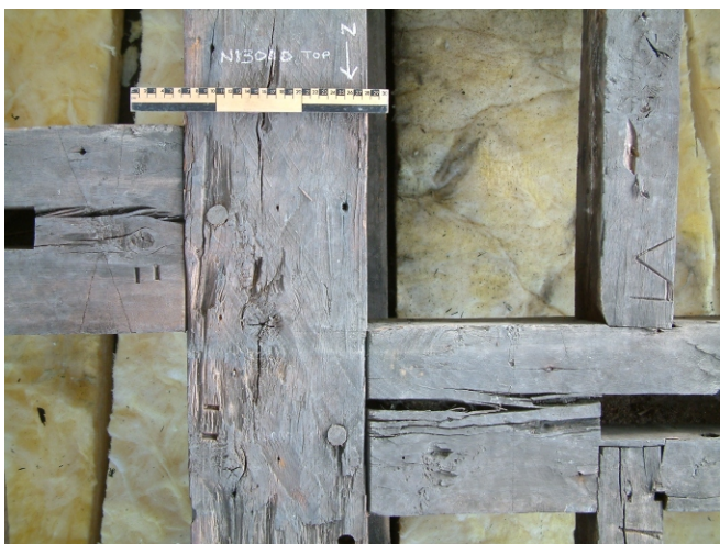
D: Marks where purlins P6 (rhs) and P7 (lhs) meet principal rafter PR6
