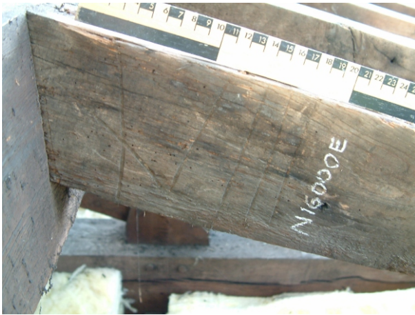
C: Race knife mark \diagdown\diagup\diagup on common rafter 6R8
