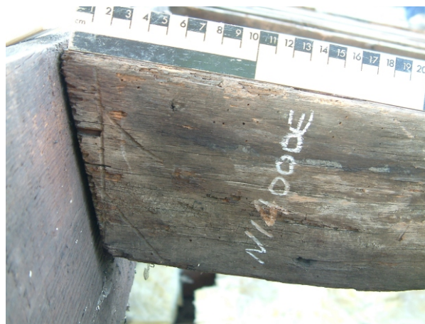
E: Truncated race knife mark \diagdown on common rafter 6R10
