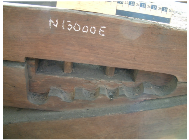
D: Empty mortice in PR6 showing moulding, slot for tenon and pegs still in situ
