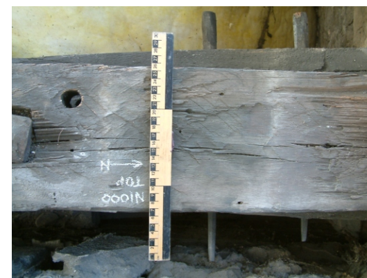
G: Intact draw pegs, points facing tower wall, indicating in situ truss construction (PR1 on Truss I)
