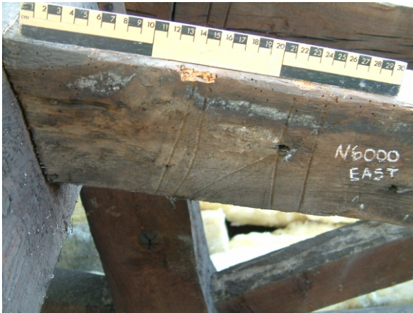
A: Race knife mark \parallel\parallel\parallel on common rafter 8R6
