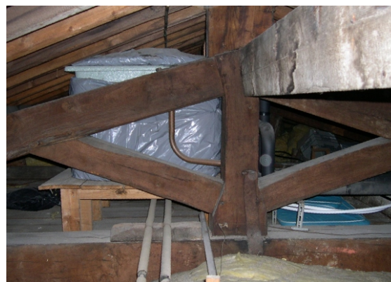
D: Master's Lodge truss showing metal strap at base and brackets securing the added block (6 th truss from tower end)
