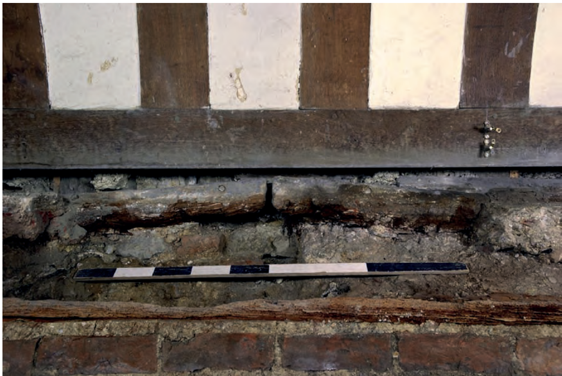
Figure 16: North wall of Fellow's Cloakroom (top) with detail of original sill beam, c.1500 (bottom).
