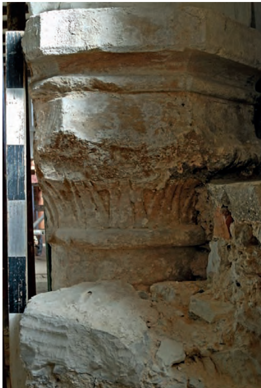
Figure 14: Details of capitals carrying chapter house vault (north pier bottom right, remainder central pier).
