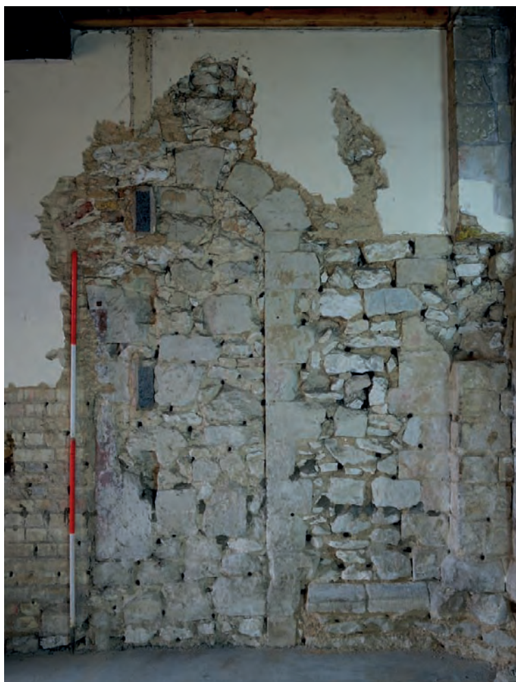
Figure 7: Doorway in north wall of Chapel prior to unblocking, with capital fragment (top right) and painted ashlar (bottom right) used in infill.
