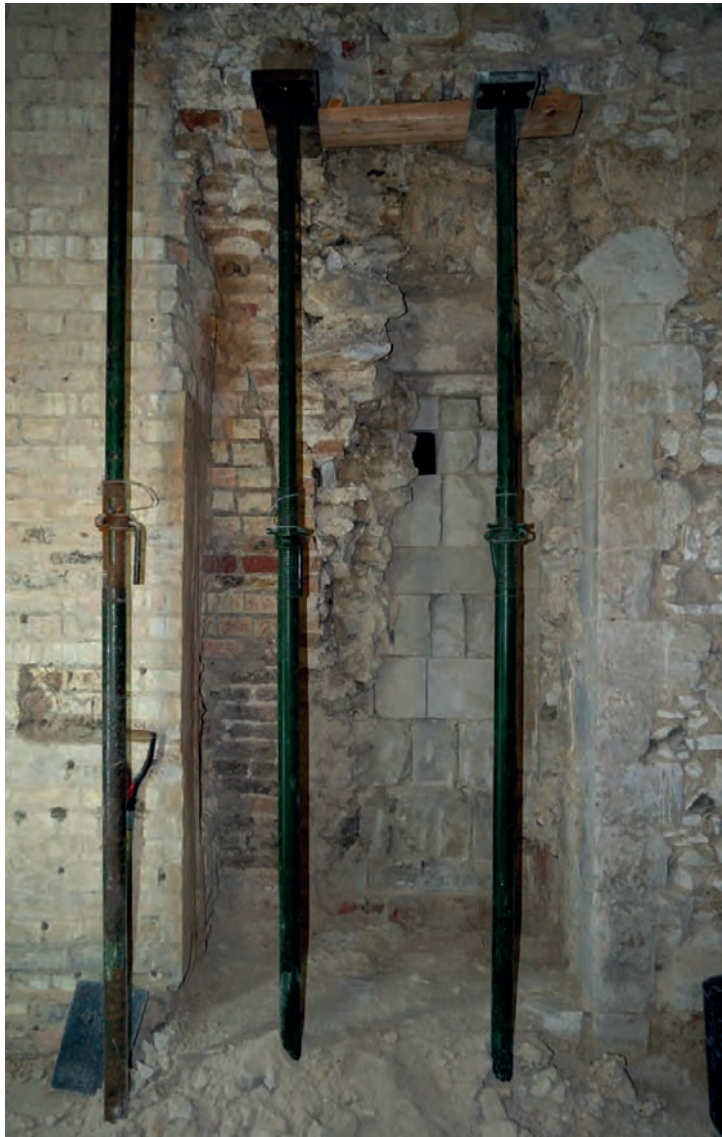
Figure 8: Doorway with original blocking removed, showing later clunch facing (left), remnants of arch recovered from infill of fireplace (top right) and the first view through the unblocked door (bottom right).
