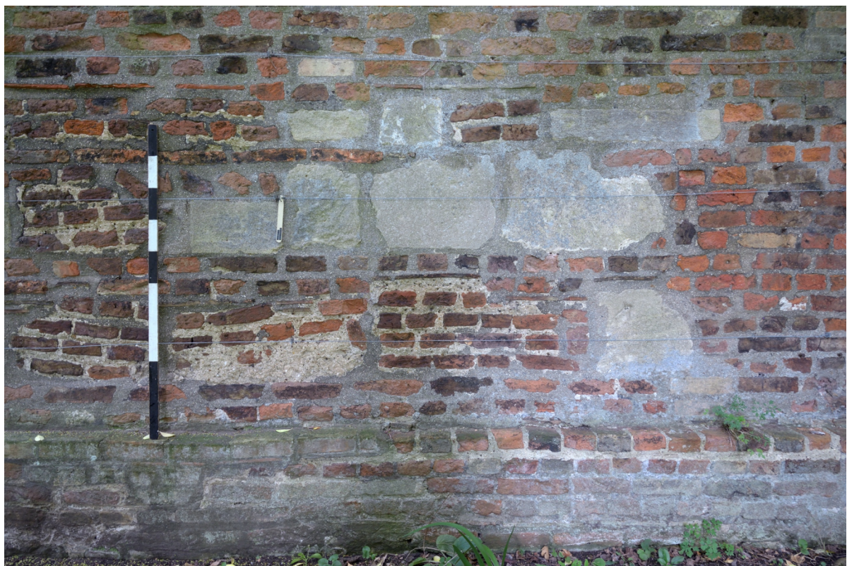
Figure 5. Elements of reused masonry incorporated into the rear elevation of the western Chimney wall (views facing east)
