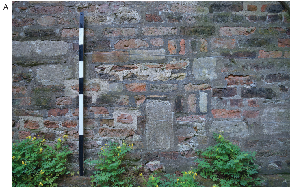
Figure 4. Photographic survey of the west-facing elevation of the west Chimney wall, with inset details showing extensive use of reused masonry and repeated episodes of repair and repointing undertaken to the fabric
