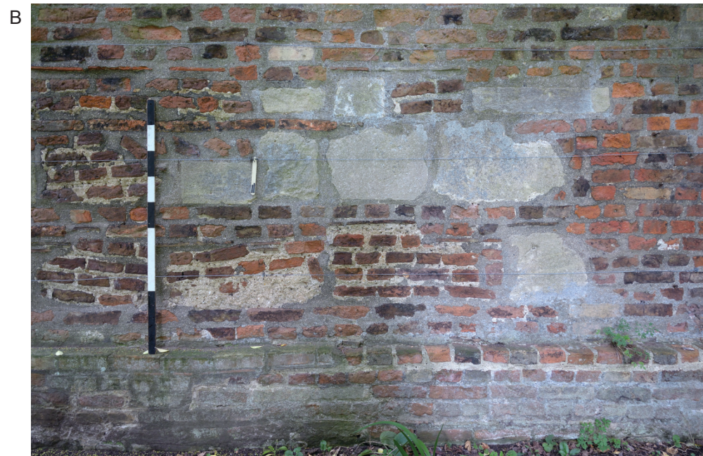
Figure 4. Photographic survey of the west-facing elevation of the west Chimney wall, with inset details showing extensive use of reused masonry and repeated episodes of repair and repointing undertaken to the fabric
